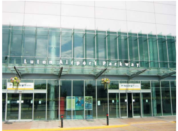
The pristine glass façade at Luton Parkway Station provides a brighter welcome for users of the station thanks to ClearShield
