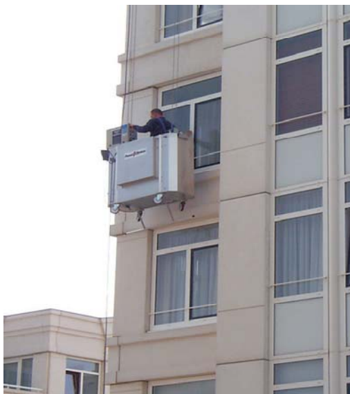
Glass treated with the ClearShield system by a Ritec specialist
