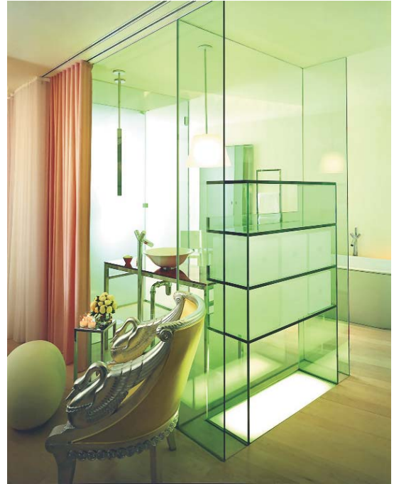
Sandblasted glass shower cubicles in 150 rooms were renovated and protected by the ClearShield System
