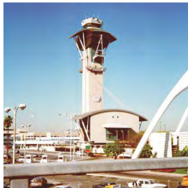
Los Angeles International, USA External glass and VCR
